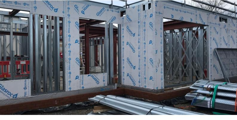
"The scheme was originally designed as a traditional RC (reinforced concrete) frame, however, following an appraisal of off-site options, Intrastack's panellised light gauge steel frame system was identified as a good solution for the project.
